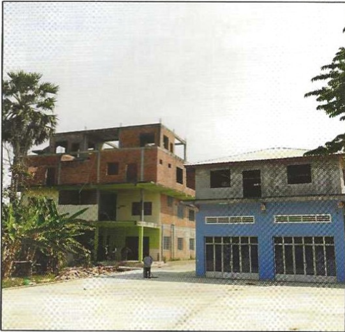
Preacher Training Center, Near Completion
